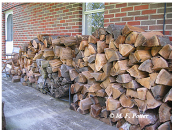
Fig. 4: Don't stack wood against the side of a building.
